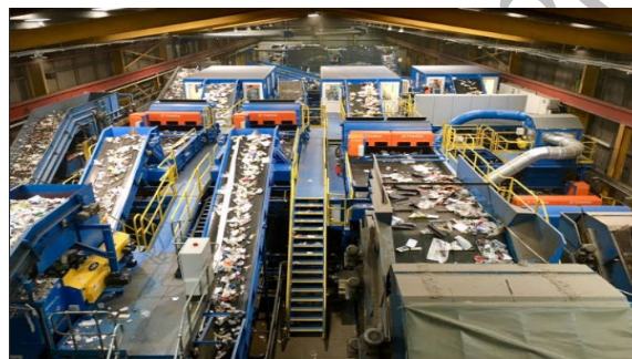
Figure F 3.2a: typical conveyor layout in waste treatment plant that requires protection under conveyors and platforms as well as protection under covered area, in addition to the ceiling protection.
